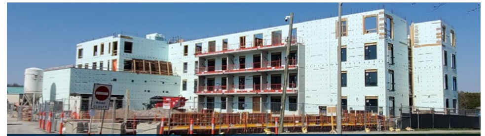
Delphine and Lloyd Martin Apartments at Parkwood.
