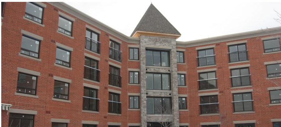
Village Housing, Lindsay: A 70 unit development with 51 affordable and 19 full market rental development with TWC as development consultant
